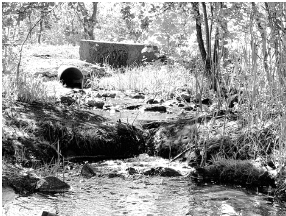
"The culvert" (Courtesy of the Mateja family)
