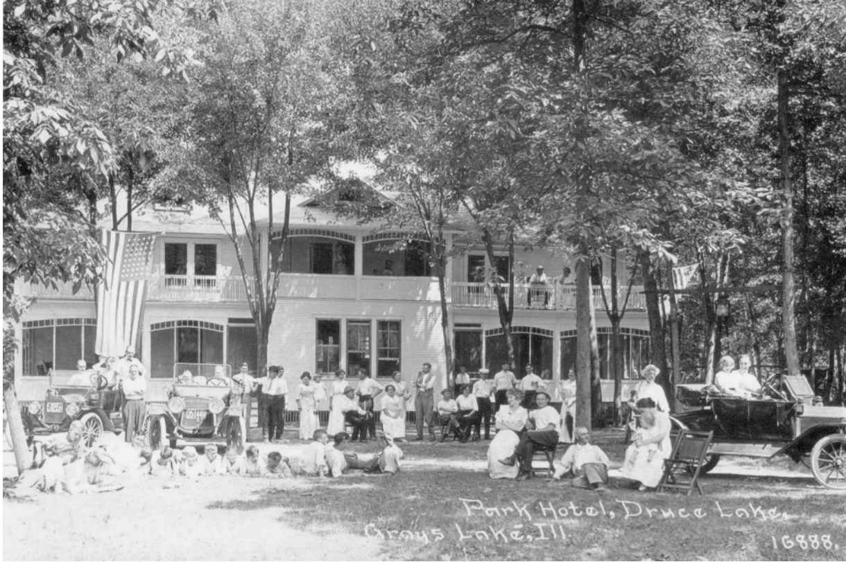
Front view of the Park Hotel circa early 1900s (Courtesy of Ted Carvis)
